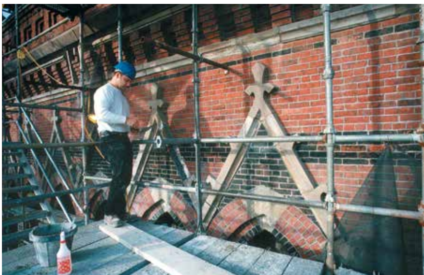
According to Dr. Judith E. Selwyn of Preservation Technology Associates in Boston, MA, the sandstone pieces with minor damage were tooled back to a new surface.
