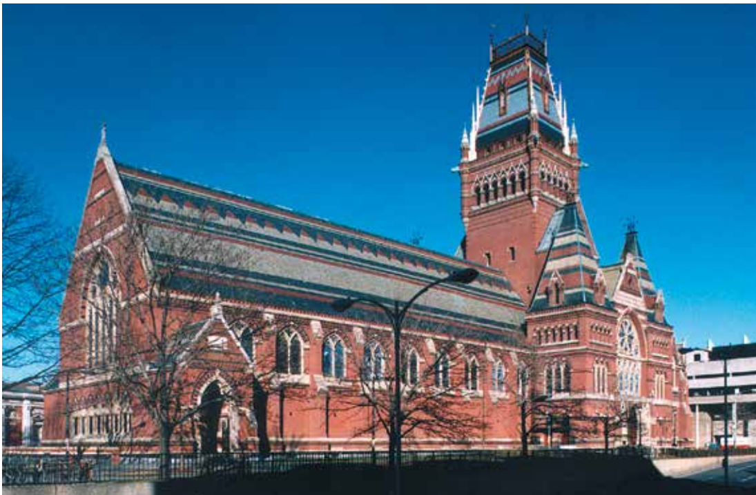
Combining North Country Unfading Black, Unfading Red, and Unfading Green slate with buff-colored sandstone, the Memorial Hall tower at Harvard University was restored to its original 1870s appearance.
