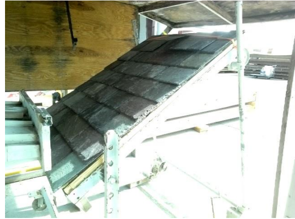
Deck #2 Before Start
