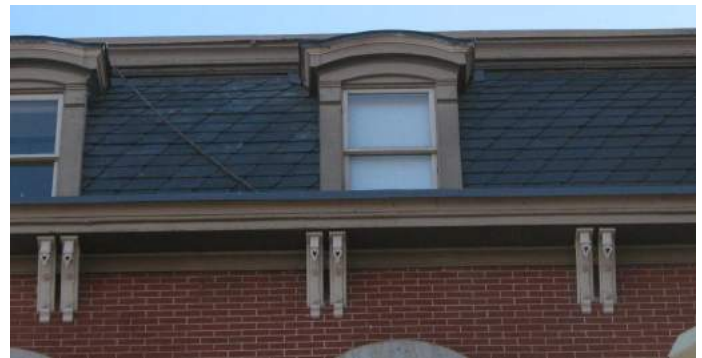
Figure 10: View of right-handed, Dutch Lap slates.
