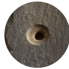
Figure 3: Drilled and counter-bored nail holes in a 100-year old slate from the Monson, Maine, district.
