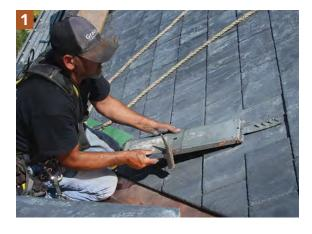
slate in place. We also use slate hooks to fill in the slates where the roof jacks were. After removing the jacks, we drive the spikes that held them so they're flush with the sheathing (2). Then we drive a black anodized, stainless-steel slate hook into the joint (3). We slide the slate under the slates above and down into the hook, which holds it in place (4).
