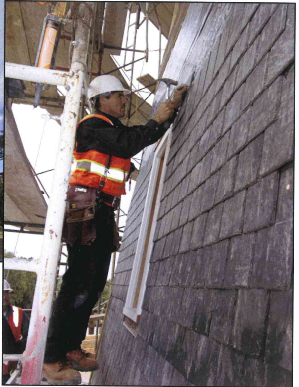
NEW SLATE ROOFING SHINGLES WERE INSTALLED ON THE WINDMILL AND COTTAGE.
