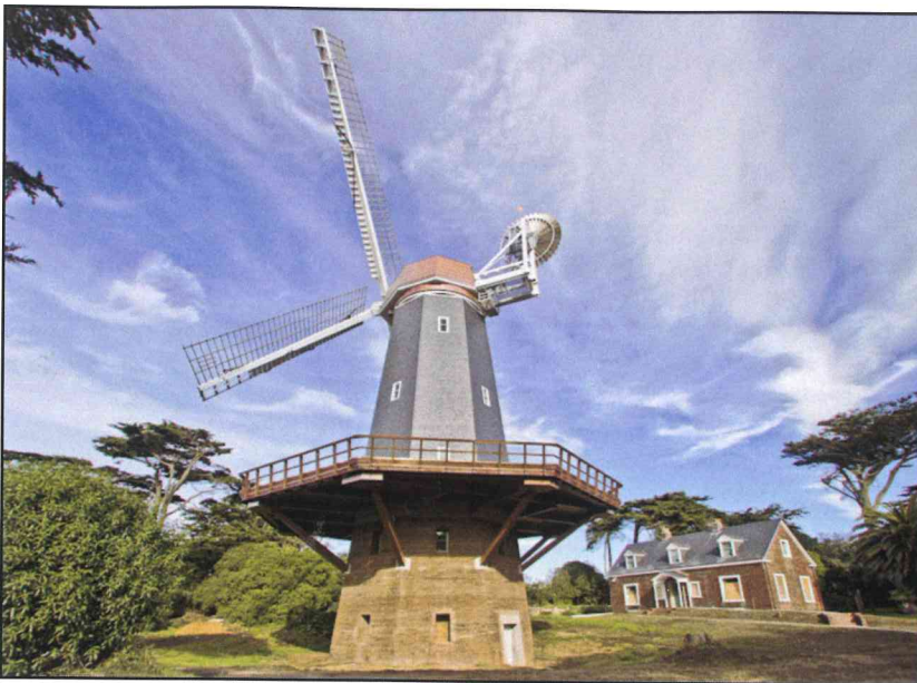
NEW SLATE ROOFING SHINGLES WERE INSTALLED ON THE WINDMILL AND COTTAGE.
