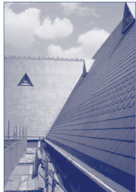
Roof over sanctuary
