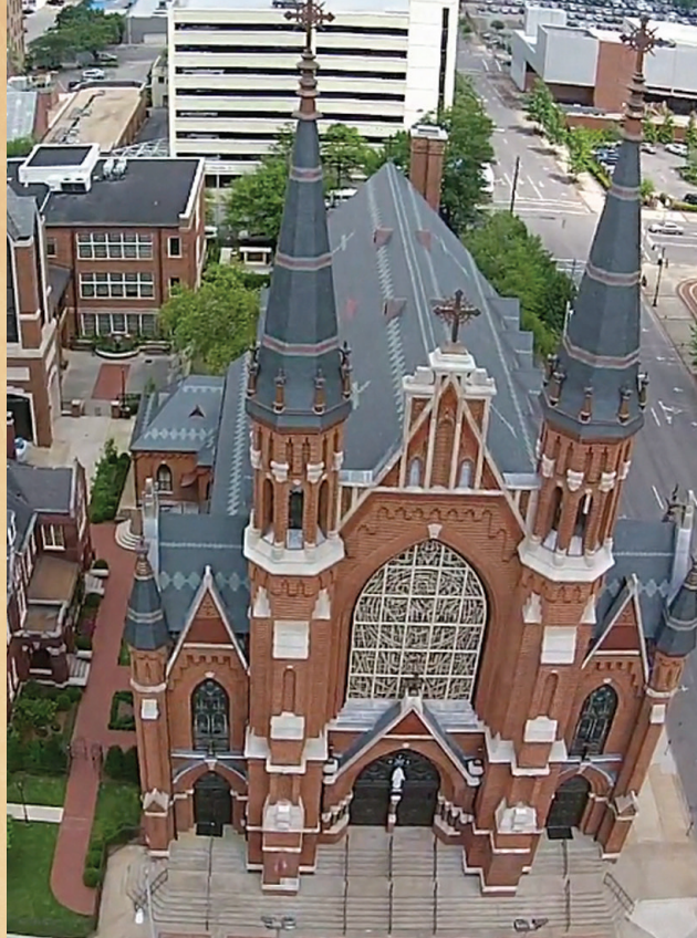
An aerial view of The Cathedral of St. Paul's newly restored slate roof system
