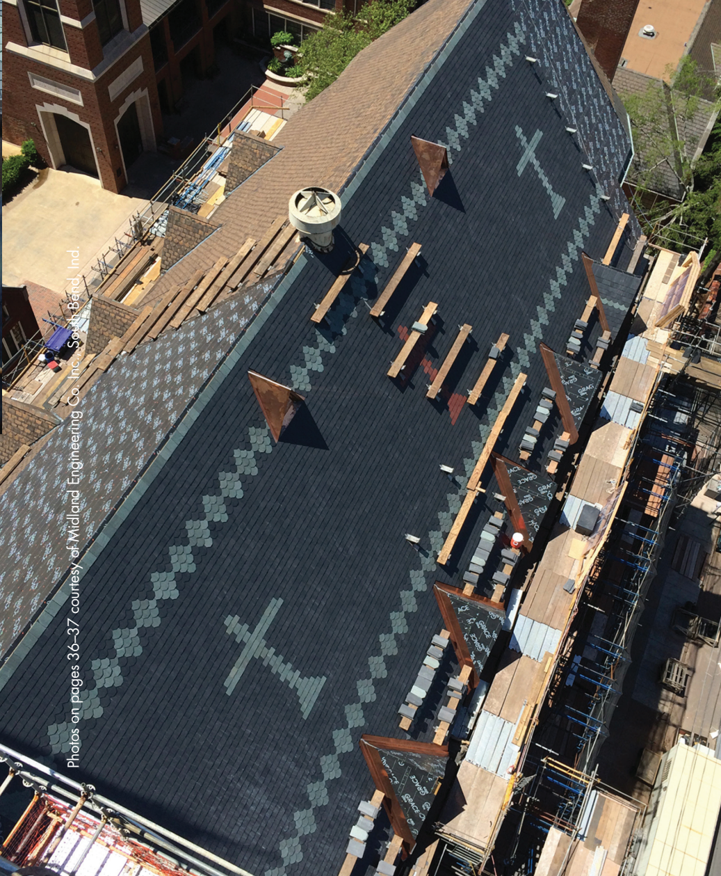
Intricate slate tile patterns incorporated three colors, six large crosses and multiple accent patterns.
