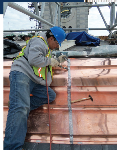
New copper cornice being installed
