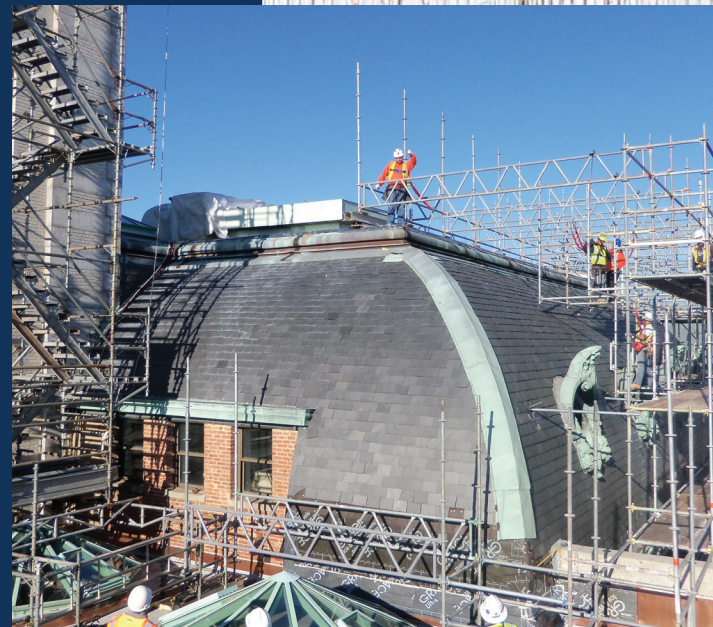
View of multiple roofs and details, including mansard slate, suspended scaffolding, hip metal and dormers
