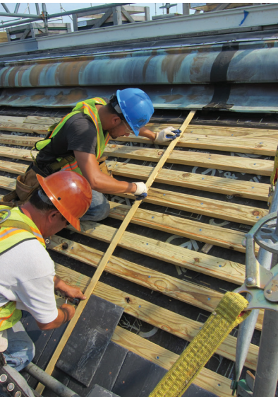
Slate on the mansard roof was installed onto wood nailers, which were preplanned and laid out so the nail holes for the slate aligned with a nailer.
