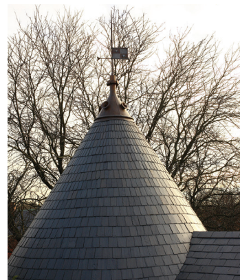
Top to bottom: While removing the slate from Edith Memorial Chapel, crew members found pieces of slate and copper with etchings that included dates from workers who originally installed the roof system in 1895; each piece of slate on the Kennedy house's cone-shaped roof was custom-cut to form the curves.
