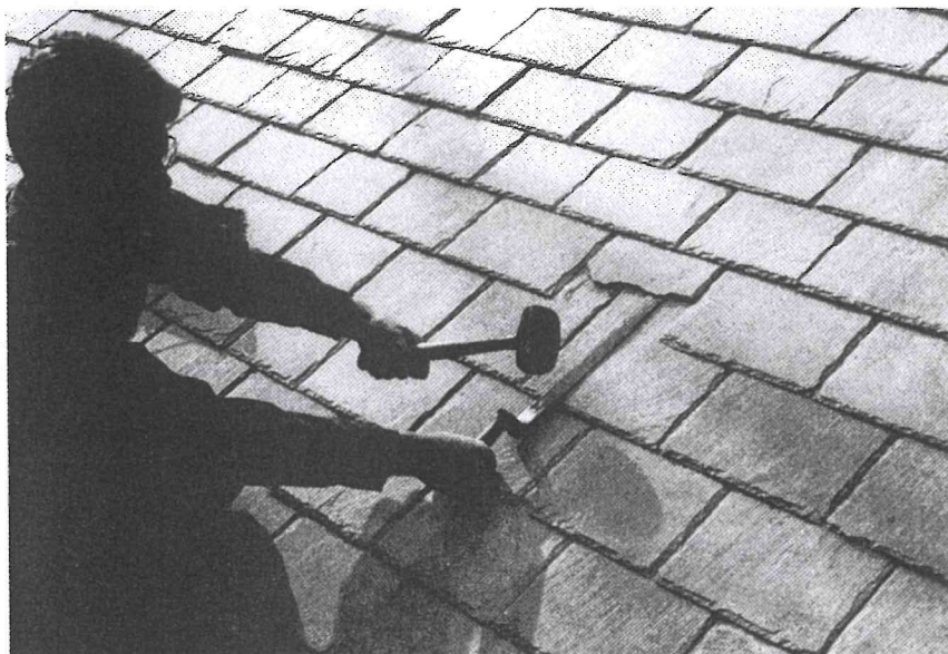
Then hammer downward on the ripper to cut or pull the nail.
