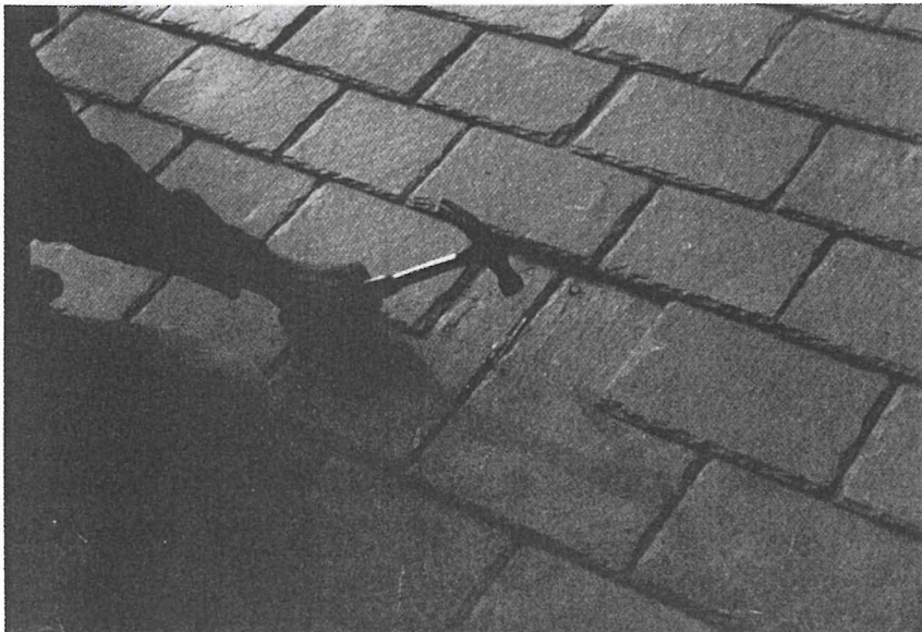
Next drive in a slate hook to hold the replacement slate.
