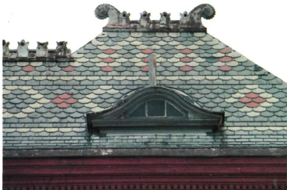
85* Base flashing above eyebrow window and cap or counter flashing below. Note also rusting galvanized iron ridge pieces
