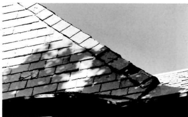
77 Slate hips: (from top) fantail, mitered, saddle
