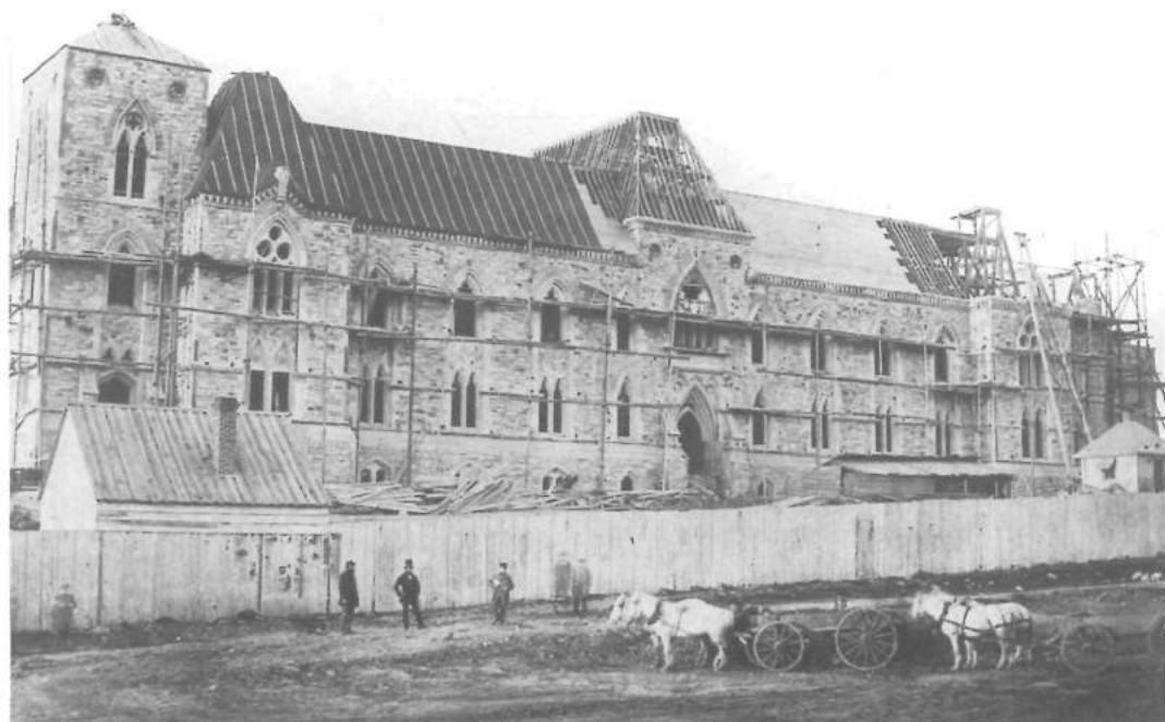
82 Felt over board sheathing of West Block, 1860s. ( National Archives, C-7715 )
