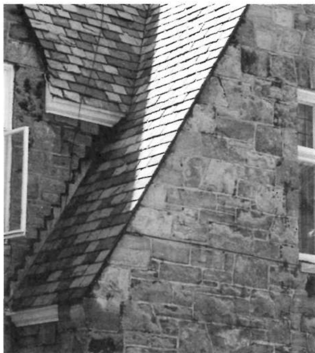
84 Base flashing running under slate
