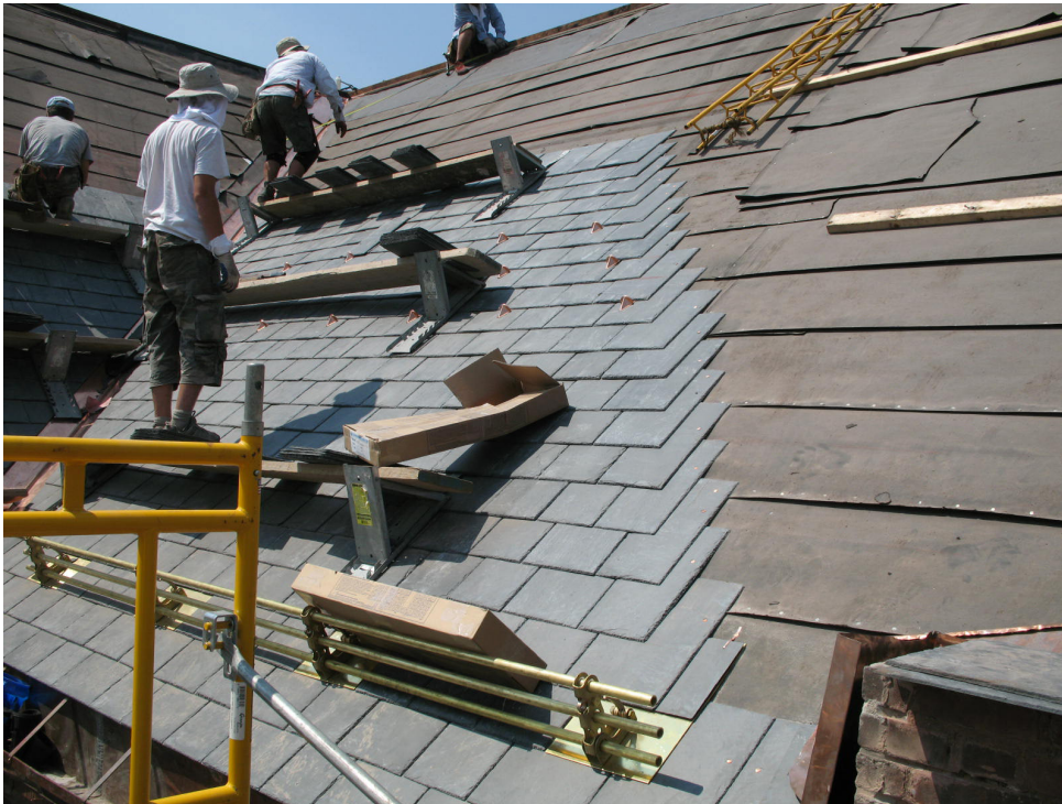
Figure 3: Slate roof installation in progress.
