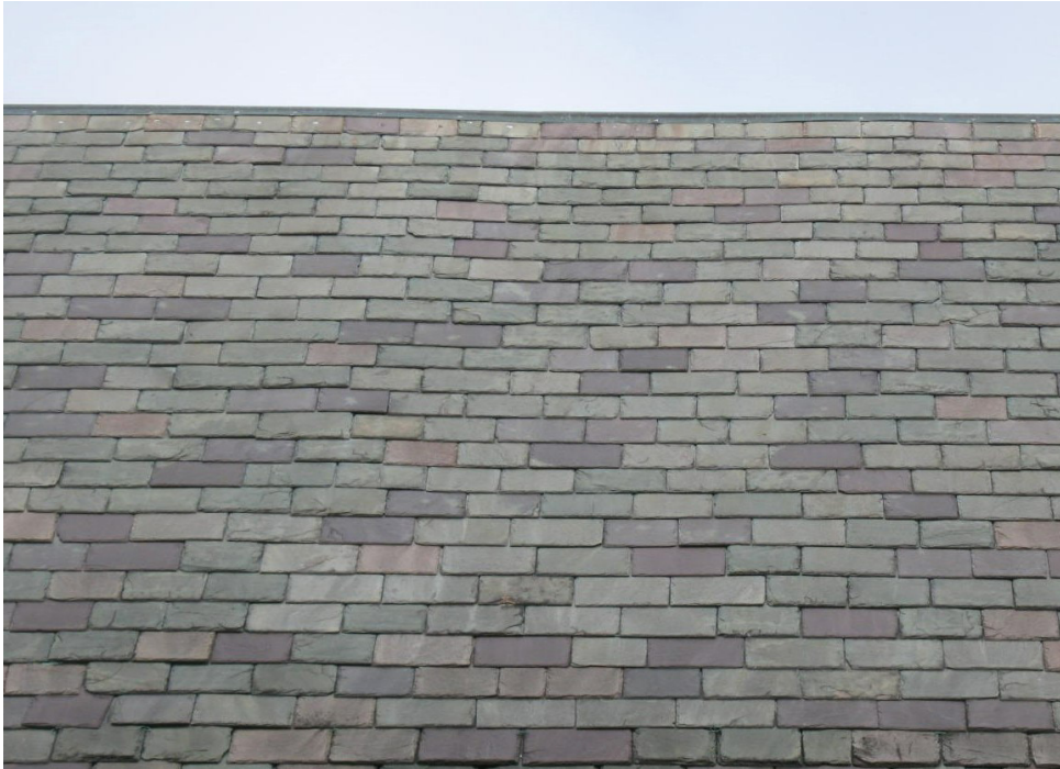
Figure 4: Example of 97-year old Vermont semi-weathering green slate mixed with Vermont unfading purple slate.
