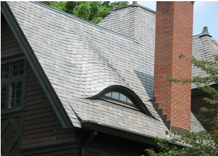
Figure 6: An eyebrow dormer covered with Vermont semi-weathering green slate.
