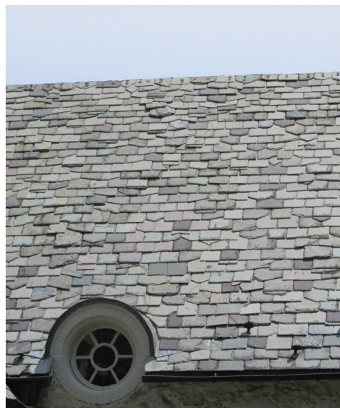
Figure 6: An eyebrow dormer covered with Vermont semi-weathering green slate.
