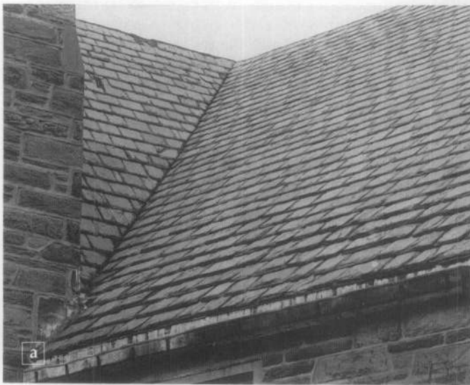
Figure 9. Valleys are formed at the internal angle of two roofing slopes. Flashing is often placed under the slate to increase moisture protect at this vulnerable joint. Shown in (a) is a closed valley where the slates are held tight to the valley line. (b) illustrates of a round valley where the transition between the two slopes is a continuous curve. It requires careful workmanship and an experienced roofer.
