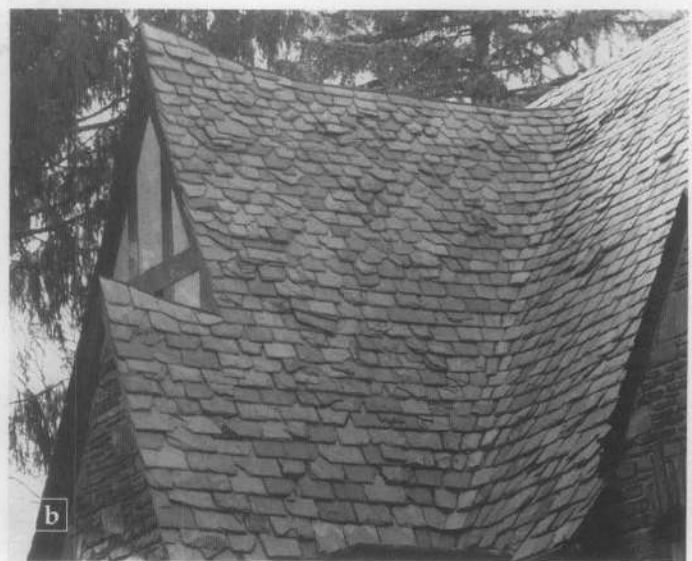
Figure 9. Valleys are formed at the internal angle of two roofing slopes. Flashing is often placed under the slate to increase moisture protect at this vulnerable joint. Shown in (a) is a closed valley where the slates are held tight to the valley line. (b) illustrates of a round valley where the transition between the two slopes is a continuous curve. It requires careful workmanship and an experienced roofer.
