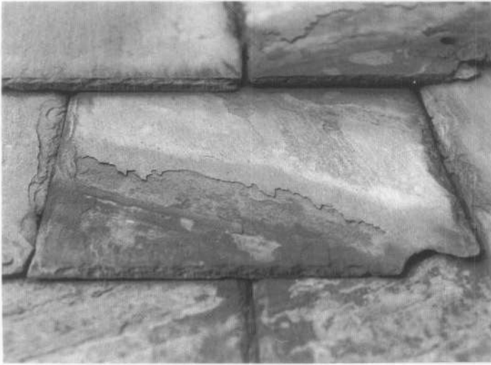
Figure 13. Paper thin lamination can be seen flaking off of this weathered, 120 year piece of Pennsylvania Hard-Vein slate.
