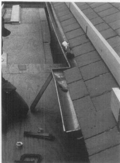
(i) Although the gutters and snow boards were the last elements installed, their support brackets were installed as the slates were laid.
