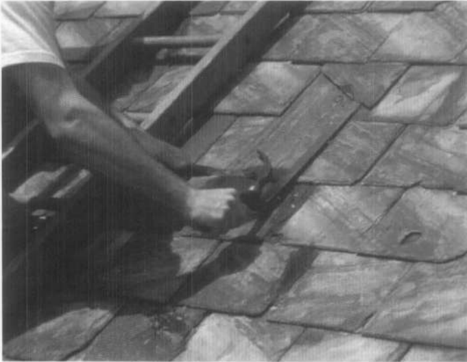
(a) A ripper is used to remove the nails from the deteriorated slate.
