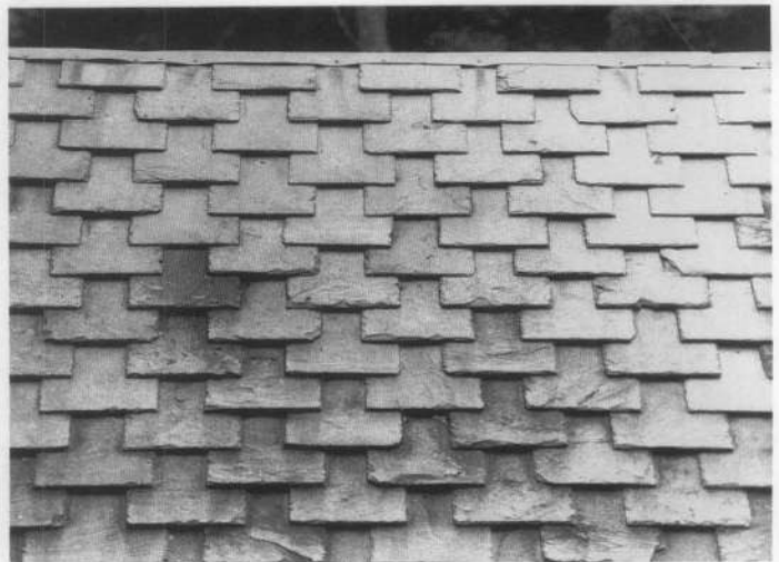
Figure 4. Widely spaced open slating was often used on utilitarian structures where ventilation was desirable. It provided an interesting texture and visual pattern to often plain structures.
