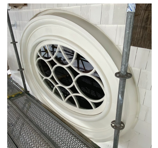
A newly renovated window
