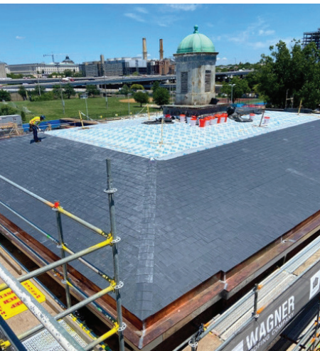
New slate roof system under construction
