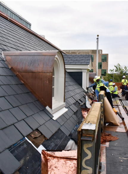
Wagner Roofing craftsmen fully restored 12 dormers.
