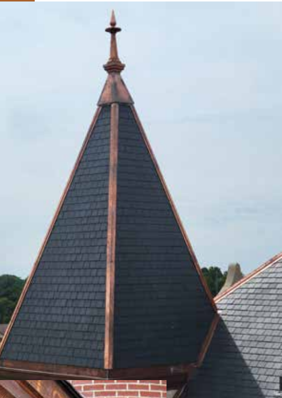
Above and left: All copper elements were fabricated by Renaissance Historic craftsmen.
