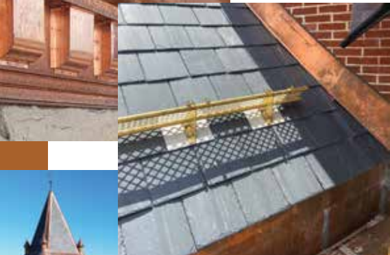
Above: Snow guards were incorporated into the roof system.
